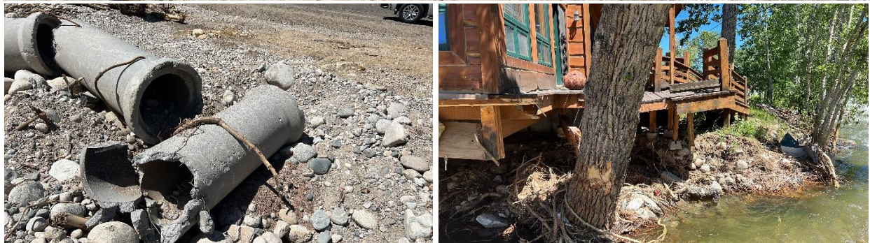
Figure 3.78: Residential Structure at Broadway/19 th Street W, at the time of the GEER team visit (45.179494, -109.246217)
