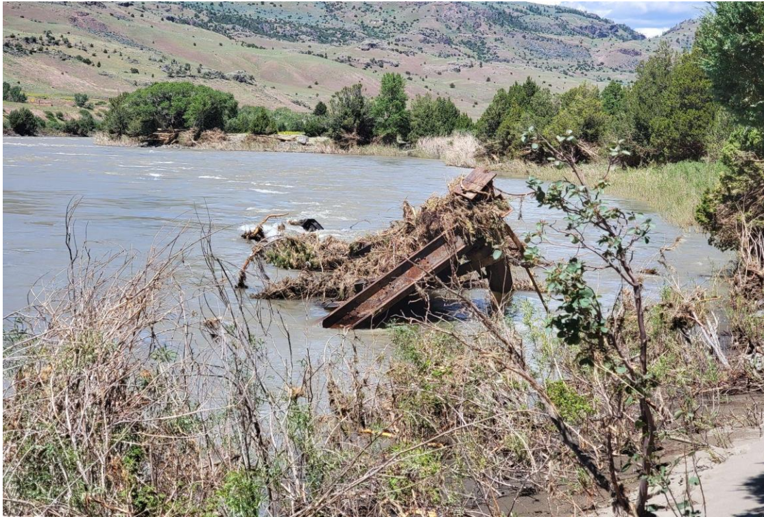
Figure 3.16: Bridge deck pieces of the Carbella bridge in the Yellowstone River
