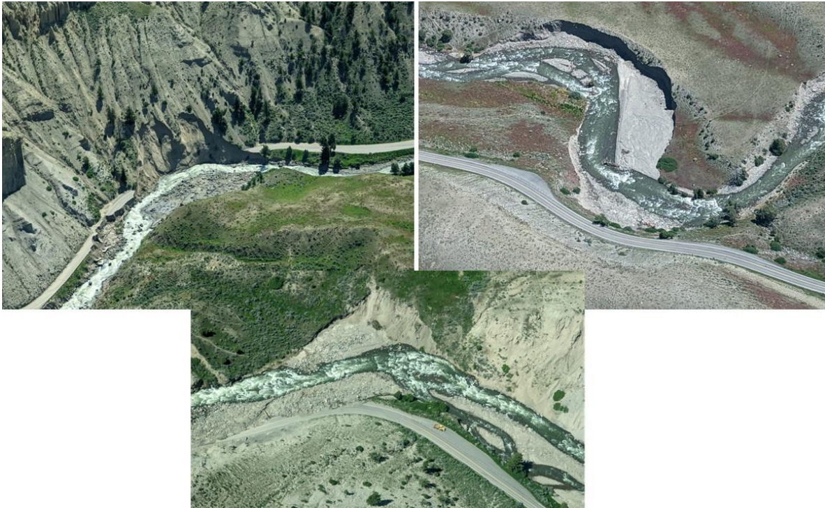
Figure 3.58: Aerial images of road failures, erosion, and slope failures near the Gardner River (Top left photo: 45.005255, -110.691759, Top right photo: 45.023285, -110.698620, Bottom photo: 45.016004, -110.692658)
