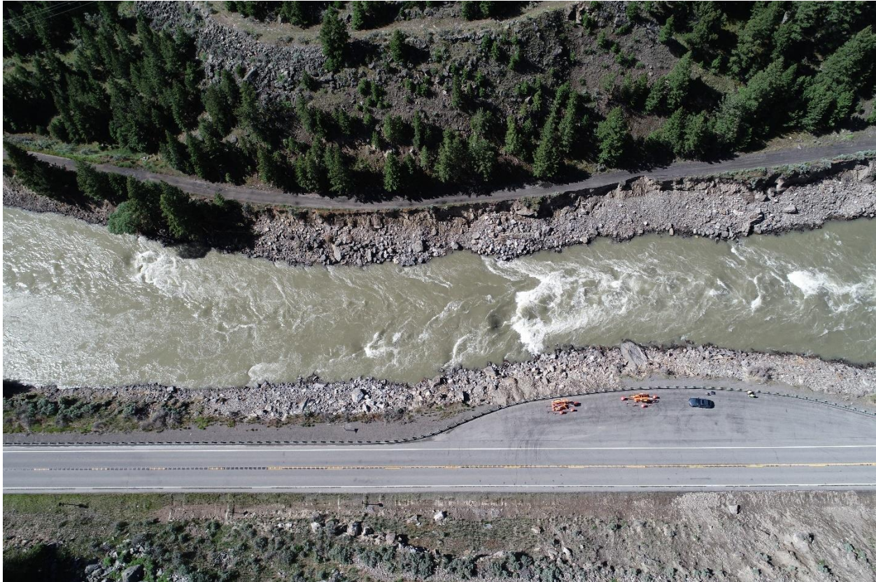
Figure 3.25: Rock Erosion along Highway 89 near Sphinx-Creek and Yellowstone River confluence (45.17018368, -110.86630538)
