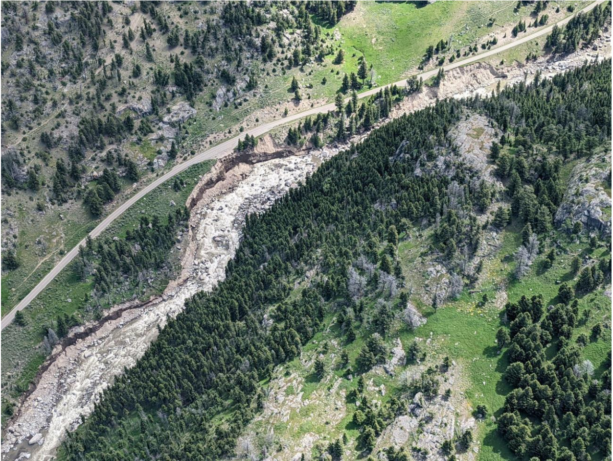
Figure 3.61: Initial meandering of the river approaching road sections (44.953619, -110.074767).
