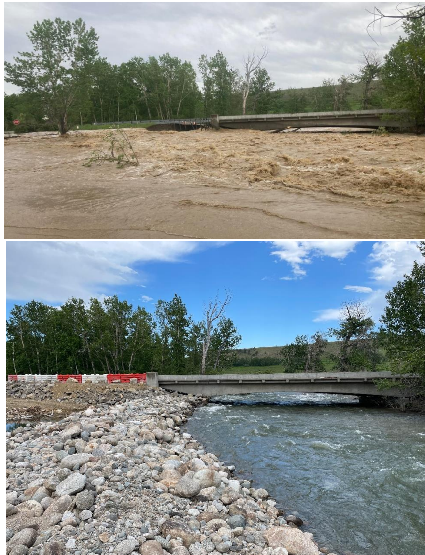
Figure 3.103: HWY 78 bridge across East Rosebud Creek in Roscoe during (top) and after the flood event; Source for top photo: https://nbcmontana.com/news/local/montana-national-guard-assists-with-search-rescue-efforts-amid-flooding ; (45.35073, -109.4955034)
