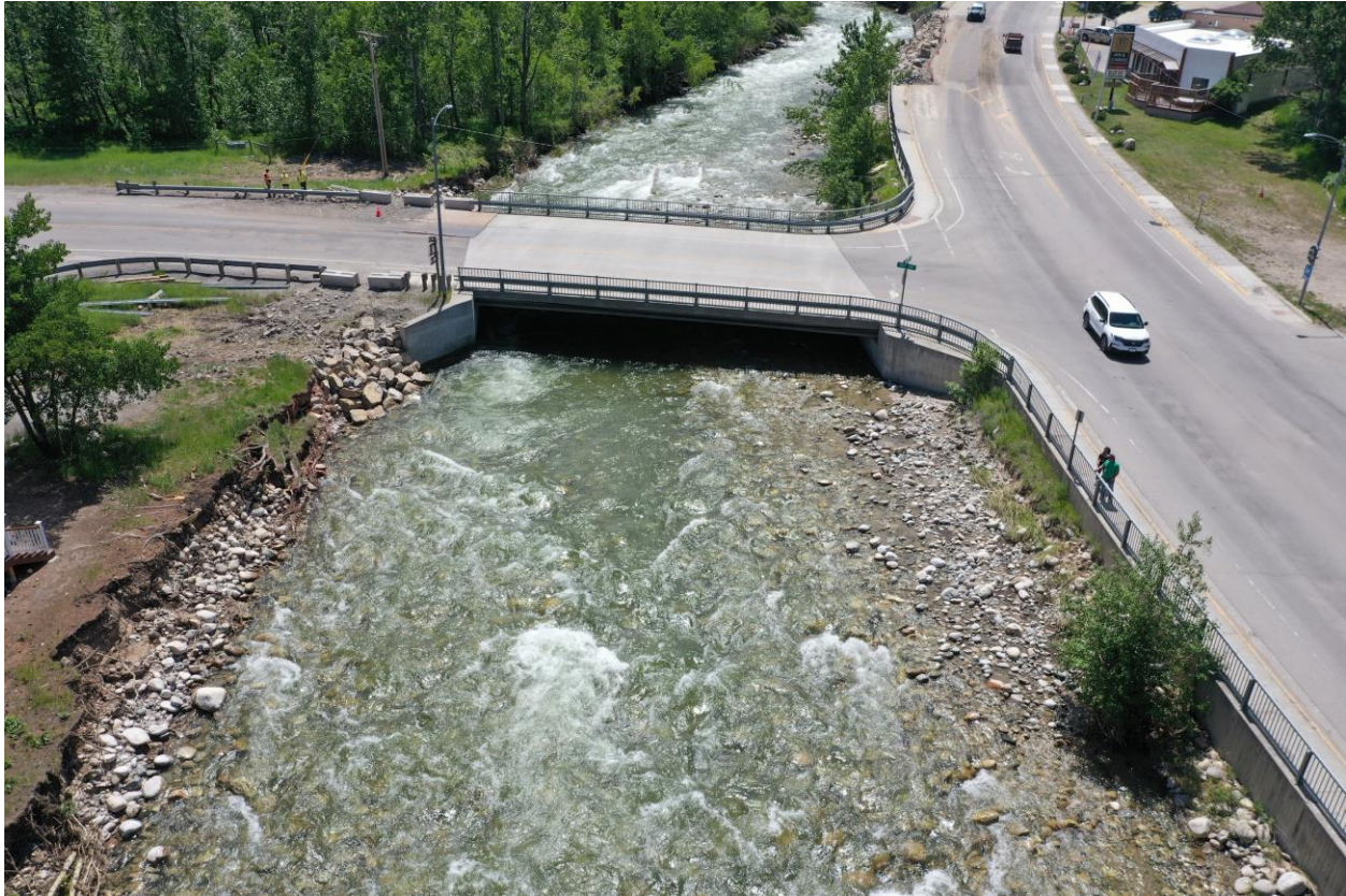
Figure 3.86: UAV image of the Montana Highway 308 bridge in Red Lodge (45.1739 N 109.2500 W)
