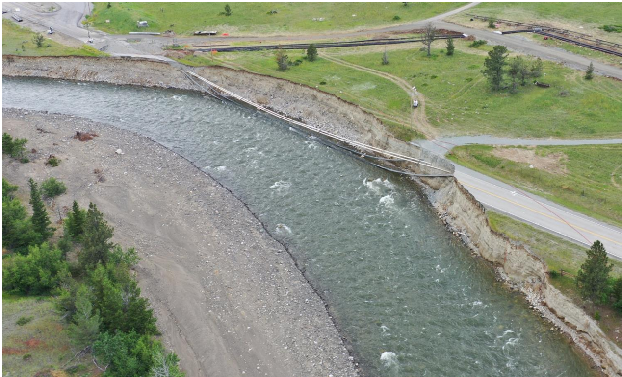
Figure 3.114: Major erosion immediately below the Mountain View Mine on the Stillwater River. Approximately 300-m of road has scoured away, with a scarp approximately 20-m high. Ductile utility lines can be seen suspended above the river. The historic channel appears on the left as a gravel beach (45.39317N, 109.87111 W).
