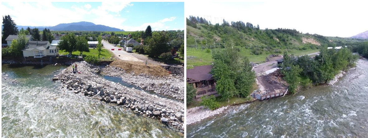
Figure 3.94: Photographs of bridge abutment and onramp area of former 9th Street bridge. (45.1889 N 109.2428 W)
