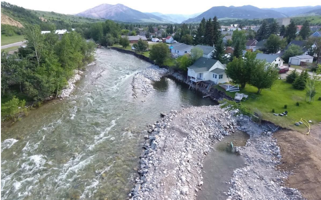
Figure 3.84: Erosion cuts and washouts along the Rock Creek River leaving substantial damage and support loss to a residential home
