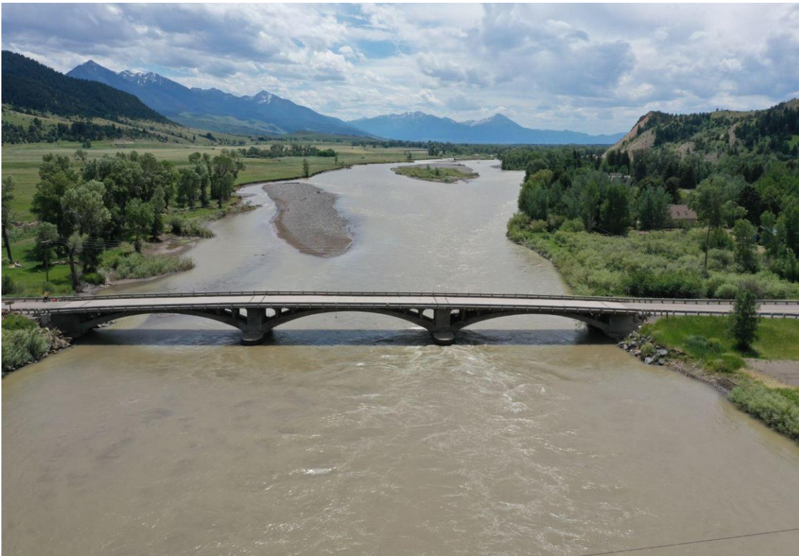
Figure 3.8: UAV aerial view of Carter bridge from downstream direction (45.59757057191095, -110.56653085768644)
