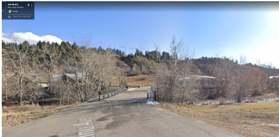
Figure 3.90: 9th Street/Kainu bridge prior to the flood (Source: google street view).
