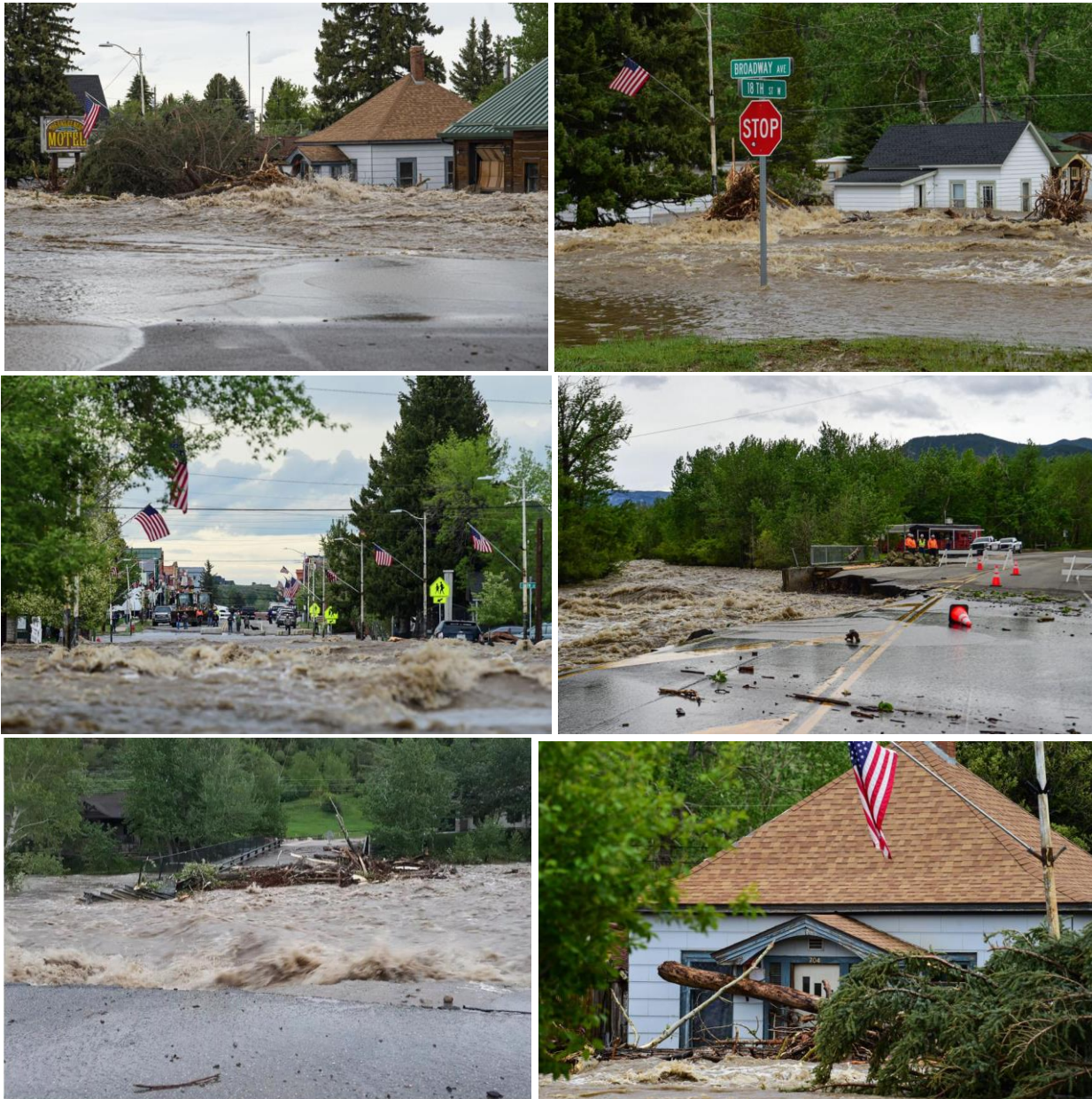
Figure 3.75: Damage in Red Lodge, MT. Source: https://billingsgazette.com/news/local/photos-extreme-flooding-devastates-red-lodge-and-the-surrounding-region/collection_d3f7e430-eb63-11ec-b484-7bd00158f809.html#26 ; Photo source of bottom left photo: Source: https://www.ypradio.org/regional-news/2022-06-20/red-lodge-area-continues-recovery-following-last-weeks-flooding , credit: Sandra Haisler
