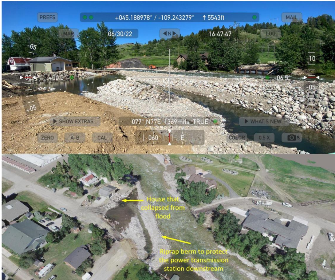
Figure 3.93: Imagery of the 9th Street/Kainu Avenue bridge in Red Lodge. Top image shows the eroded and repaired abutment; bottom image is a screenshot from the 3D UAV SfM model (45.1889 N 109.2428 W)
