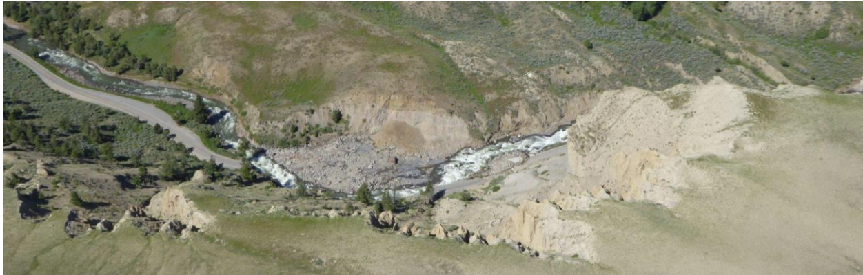
Figure 3.57: Aerial images of road damages along the Gardner River between Gardiner and Mammoth Hot Springs taken on Jul 1, 2022.
