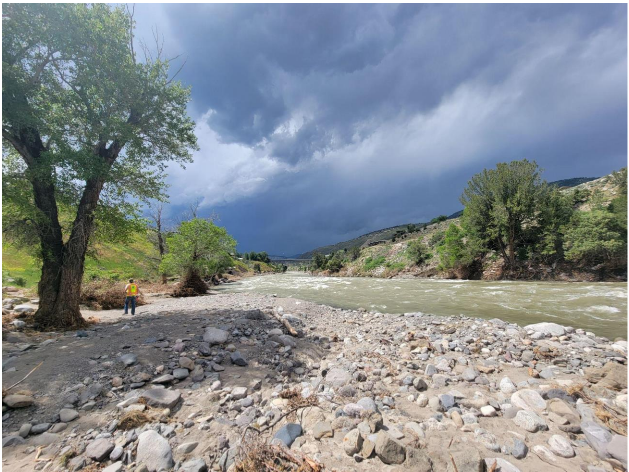
Figure 3.39: View from the confluence towards Yellowstone River Bridge.
