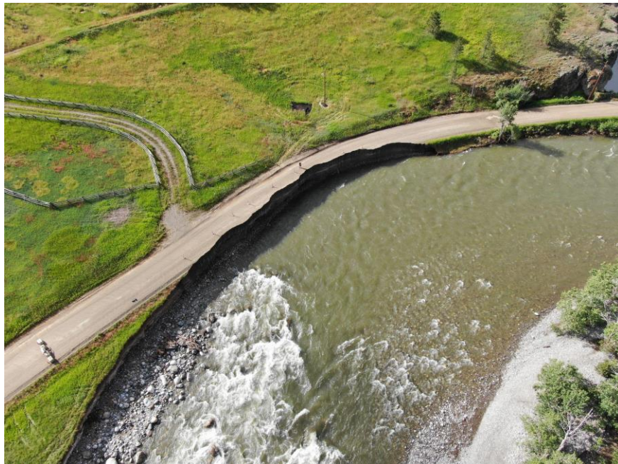
Figure 3.120: The 100-m long scour event along the Stillwater River at the Cliffswallow Fly Fishing Recreation Area (45.5108N, 109.63666W). Scarp is approximately 8-m high.
