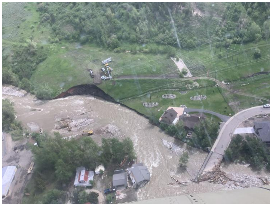
Figure 3.91: Bridge Collapse at 9 th street and large erosion failure, Source: https://www.kulr8.com/news/officials-gather-in-red-lodge-to-discuss-flooding-impacts/article_d7e3a7b2-edbd-11ec-a518-9bfe1b67d2ad.html
