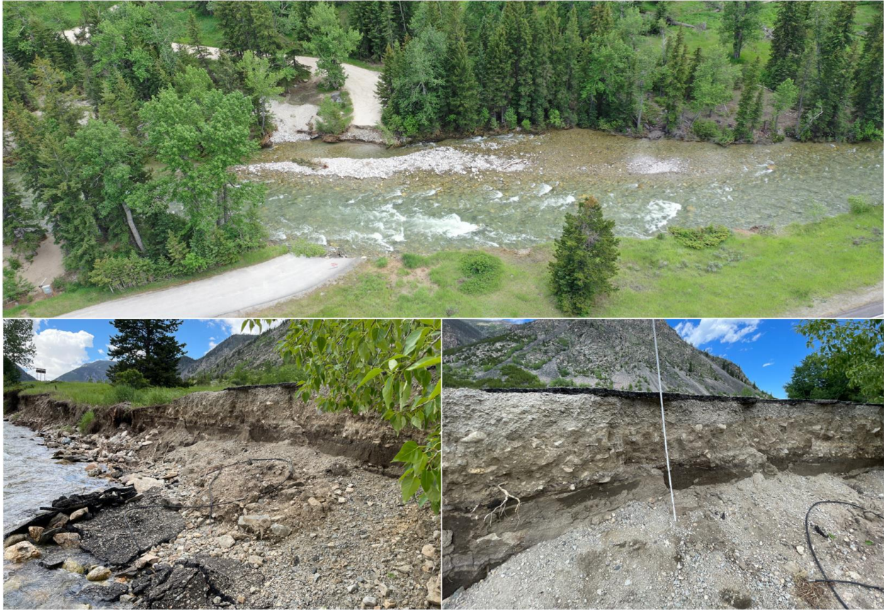
Figure 3.72: Washed out bridge at USGS Gauge Station on Rock Creek (45.086N 109.330826W).
