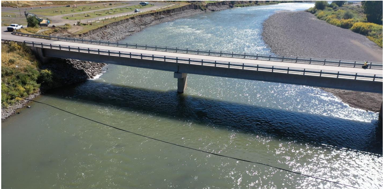
Figure 3.23: Top: UAV Image of erosion surrounding the Cinnabar basin onramp, Bottom: Aerial photo of Cinnabar bridge at the time of the team's visit (45.11185551, -110.7926037)
