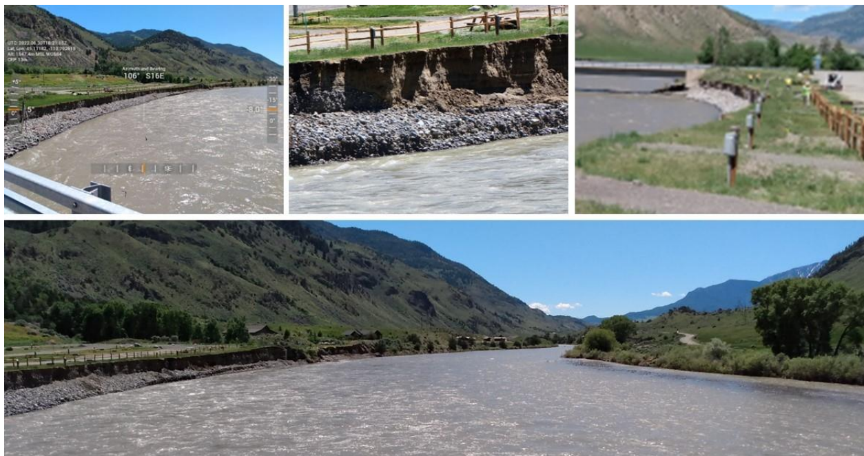
Figure 3.21: NE upstream riverbank being subject to significant erosion (45.1115243, -110.79229245).
