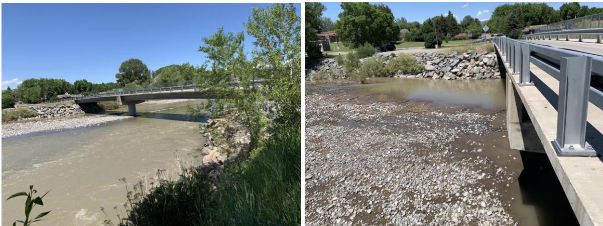
Figure 3.2: Bridge @ 9th street/Yellowstone during GEER visit. An extra span allows for the river to move between the banks and erode and deposit sediments freely. Note the new gravel bar deposited from the recent floods. Also note the “dirty” nature of the bar, indicating flow velocities were low enough for finer sediments to deposit at this bridge in the flood. (45.64970166034406, -110.56177707651814).
